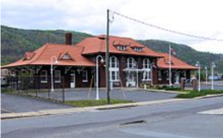
Former Clinchfield Depot in Erwin, Tennessee
